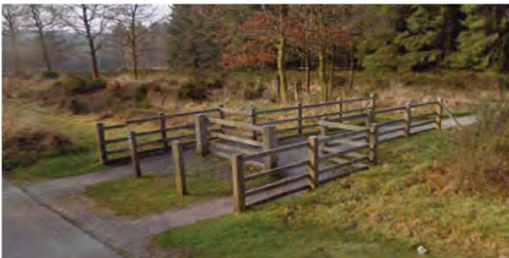
Aston Gate – 1.5m, 2 Way Suitable for mobility vehicles due to the extra strength of the bottom two rails. The two-way catch, EASY LATCH and 180 degree self closing system is suitable for users of mobility vehicles.
